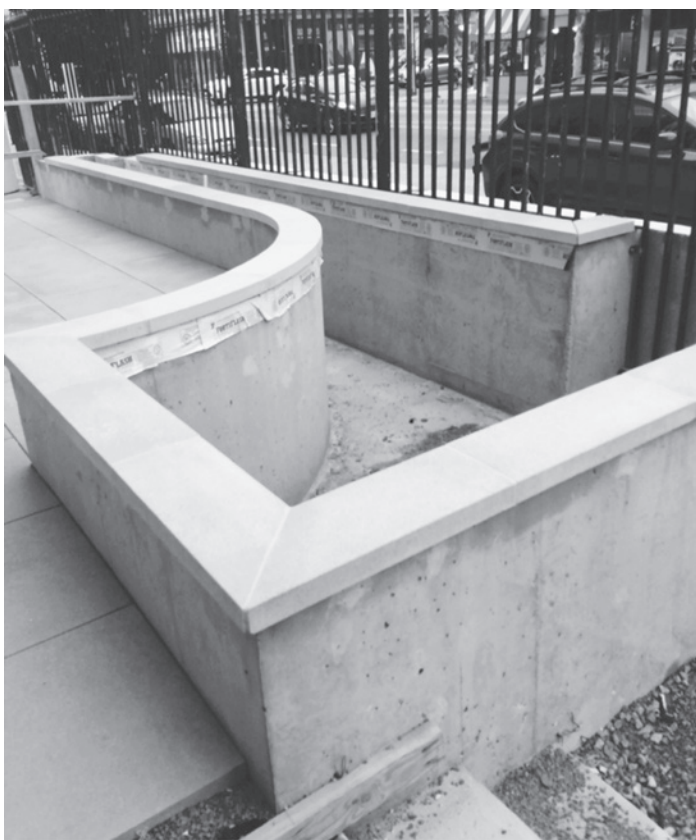
A view of the low walls along the front of the new Cathedral, which shows the work to be done. This includes facing the walls with granite, extending the pavers to the street, and placing new gates. Some of the gates will be motorized.
