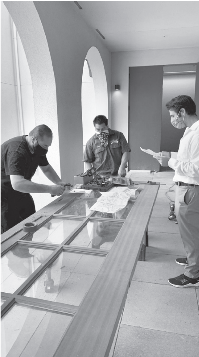
The interior door installation is in process
