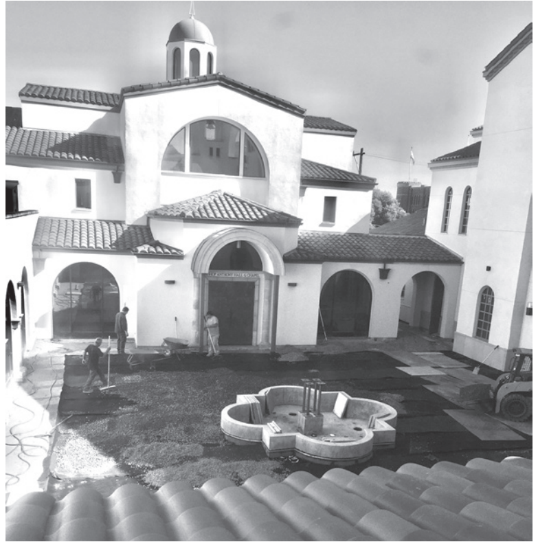
The laying of the courtyard pavers has begun. Several inches of crushed rock is being laid over the waterproofing membrane and under the pavers, to facilitate drainage. The last outdoor item which will be tended to is the Courtyard fountain.
