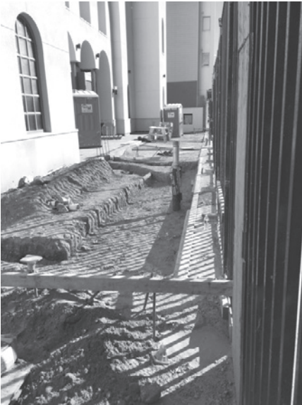
The footings along Valencia Street are being laid. This will enable the fence to be pushed back and positioned behind the new sidewalk, which will be laid as this issue of the Herald is being delivered to you.
