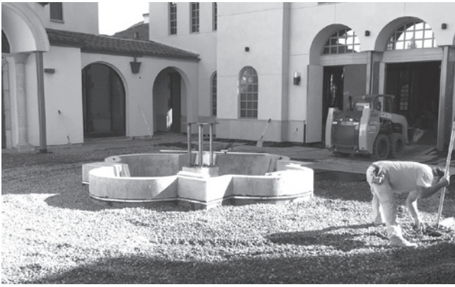
The laying of the courtyard pavers has begun. Several inches of crushed rock is being laid over the waterproofing membrane and under the pavers, to facilitate drainage. The last outdoor item which will be tended to is the Courtyard fountain.
