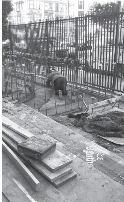
The footings along Valencia Street are being laid. This will enable the fence to be pushed back and positioned behind the new sidewalk, which will be laid as this issue of the Herald is being delivered to you.
