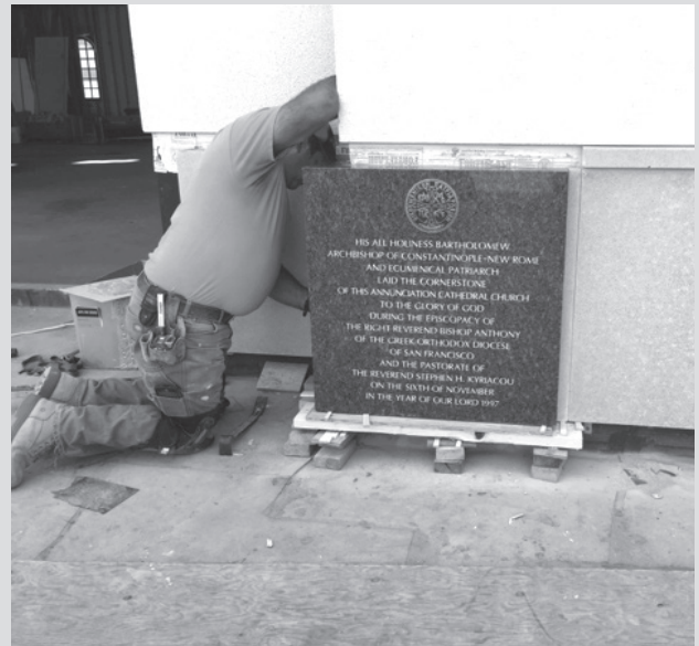
One of the workers, securing the cornerstone.
