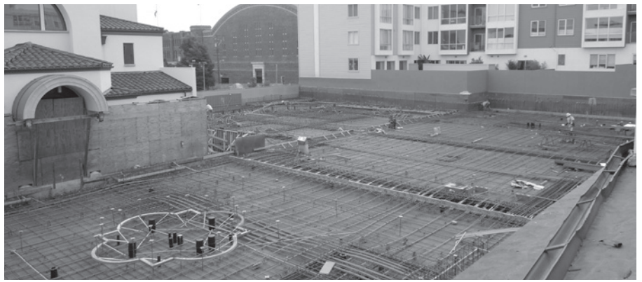
The deck is fully prepared to receive a total of about 1.5 million pounds of concrete. The first pour took place just before Christmas; the second pour will take place around Epiphany. Then, the vertical steel begins to be erected. Notice the shape of the courtyard fountain. It is modeled after the remains of the courtyard fountain of Agia Sophia in Constantinople.
