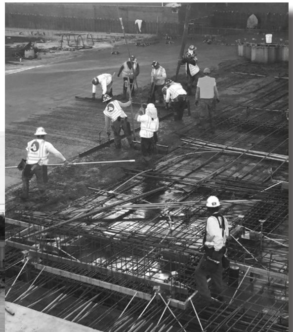
Second of two concrete pours
