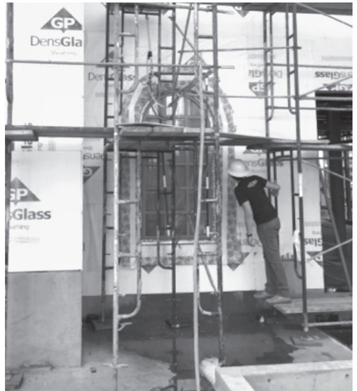
Window ready for testing
