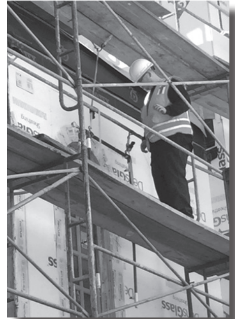
One of the 135 windows being water-tested
