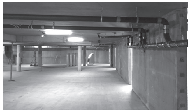
A partial view of the parking component, beneath the new Cathedral.
