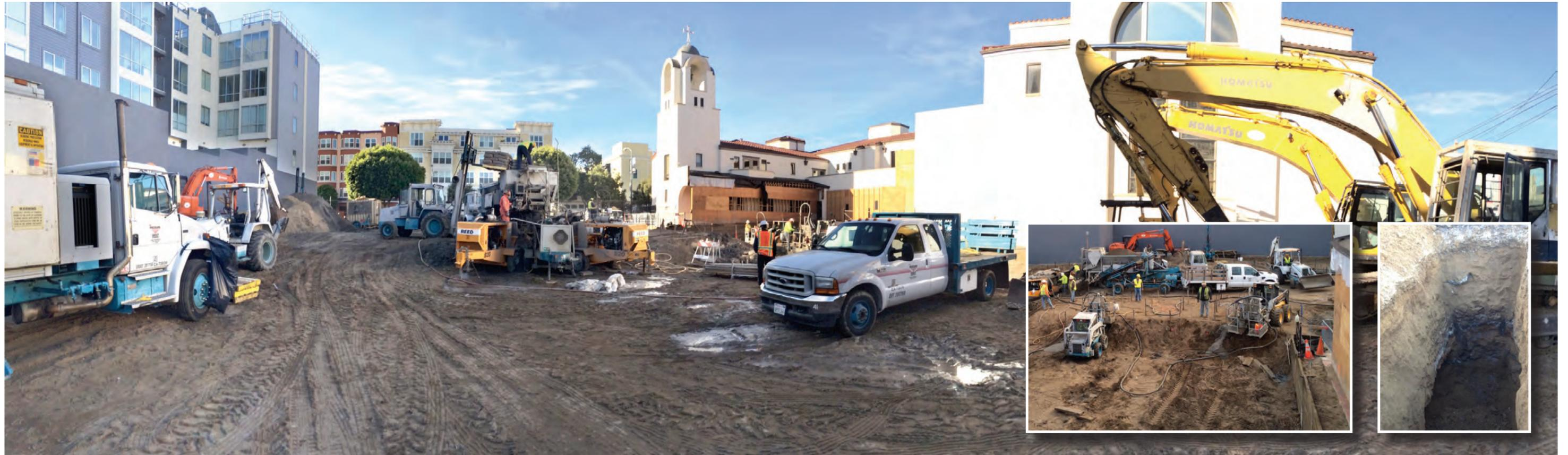
Construction of our new Cathedral is proceeding well. The shoring columns for the excavation are all installed, and some of the lagging between columns has been installed. The rest of the lagging will be installed as the excavation for the parking garage goes forward.
